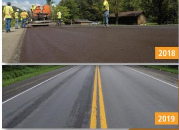
distresses. KYDOT chose this new product trial using Surface-EXT to increase the road's longevity while reducing the cracking that keeps occurring. Reduced project cost was also important to them. For little cost added to the project, they will not only add years of life with micro surfacing but will receive a high return on investment as well.
