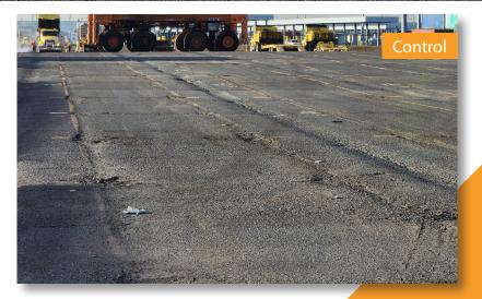
The pavement of this terminal sees severe rutting caused by container moving equipment. These extremely heavy pieces of equipment are forced to run on an exact path and cause damage to the asphalt. To **extend** the **pavement life cycle** at this facility, a control vs. fiber project was completed.
