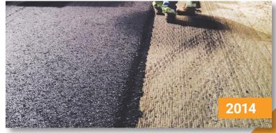
SR208 is a heavily traveled road in an Amish community that withstands not only cars, but also a large amount of horse and buggy traffic. A good portion of the road is also asphalt over brick. PennDOT 11-0 elected to mill up the road and place FORTAfied® asphalt to defer the reflective cracking and provide tensile strength to combat the rutting issue.
